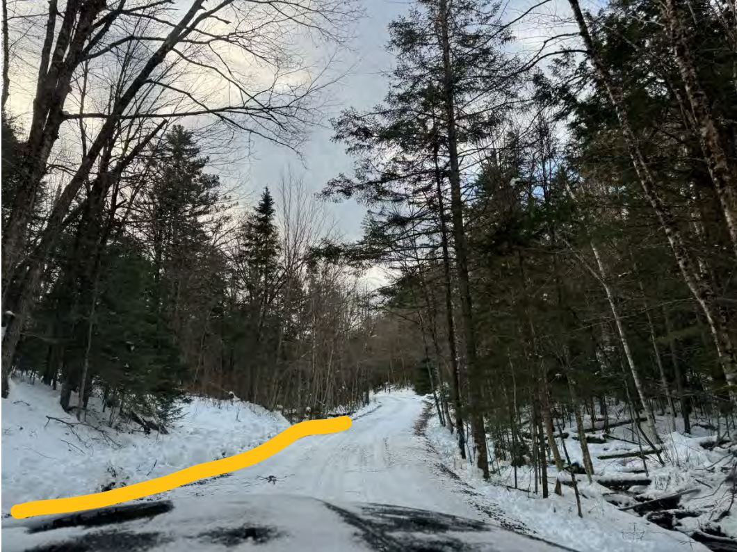
16731 before 1 - stone line ditch left side with erosion stone
