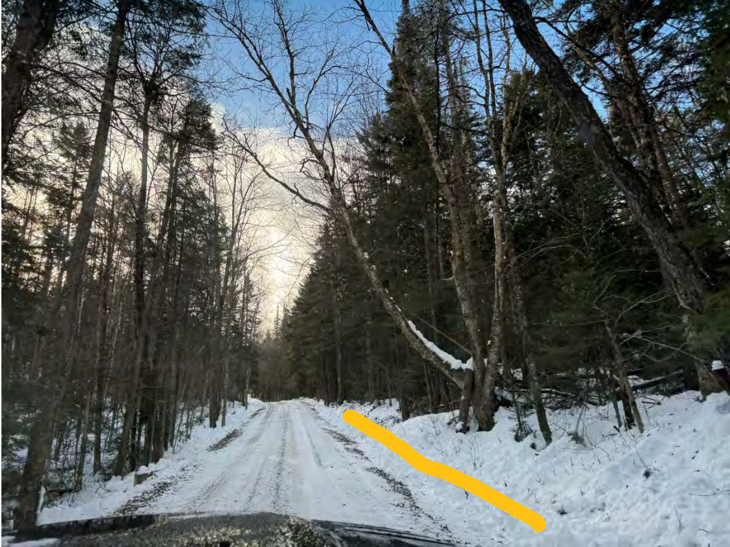
16734 before 1 - reshape and grass line ditch right side
