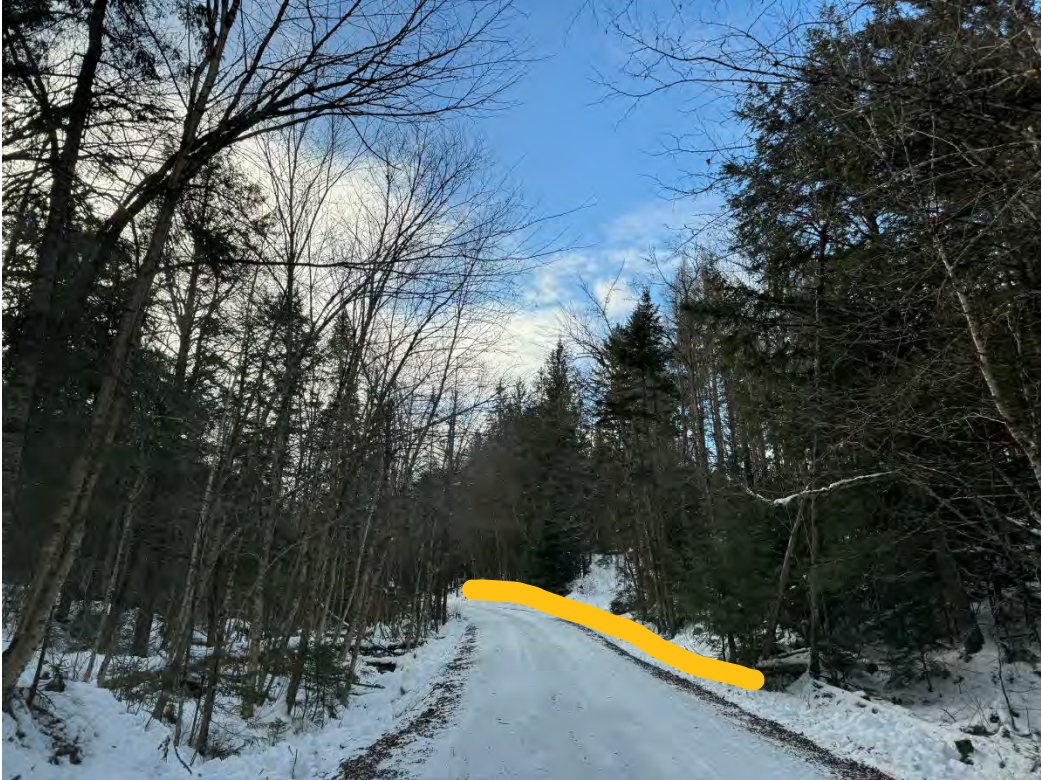
16731 before 2 – after driveway access, reshape and grass line ditch right side
