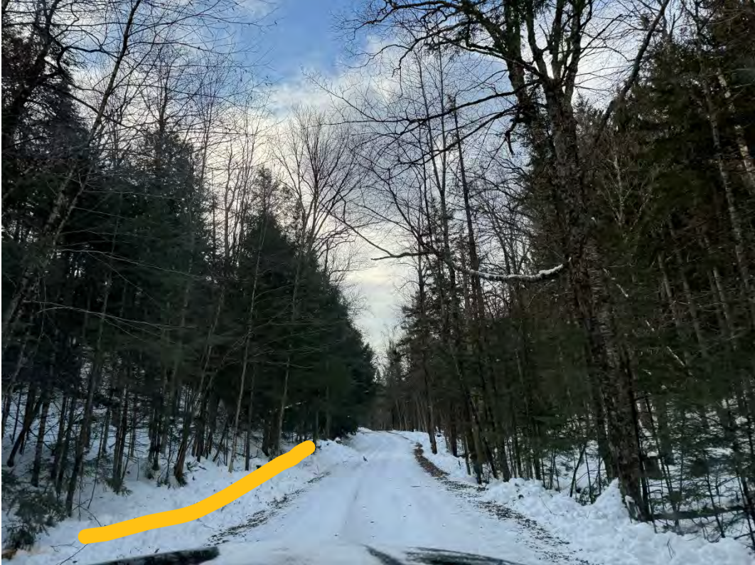
16730 before 1 - stone line ditch left side with erosion stone
